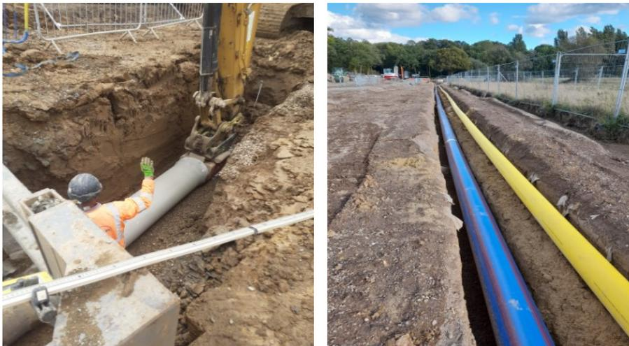
Photos on the left: Show underground drainage and utilities materials being installed.
