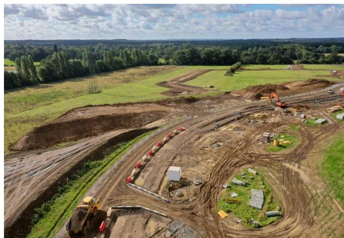
Photo on the right shows works at the junction of Park Lane/Nine Mile Ride. These works included install of new drainage systems, connection of new utility supplies to existing supplies and tie-in of the new road to the current junction. The junction was reopened at the end of October 2021.
