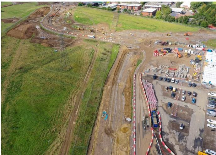
Main construction works are well underway at a number of locations across the sites, focusing initially on the bulk earthworks and drainage works as well as working with the utility companies to install and divert all the necessary services such as gas, water and electricity. As you can see, works have progressed to the extent that the beginnings of what will become the new road alignment are starting to take shape on the ground.
