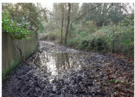
Drainage on a section of this path has been a problem for years - with blocked ditches, a blocked culvert and water running down the path.
