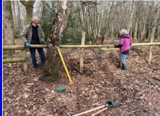
The surrounding fence had also deteriorated and plans were put in place to carry out the improvements in the Spring of this year. Suitable chestnuts were identified adjacent to the car park and new posts were cut to size. The rails were pre-cut and then delivered to site.
